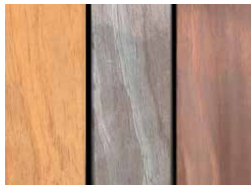
Ticari newly installed
